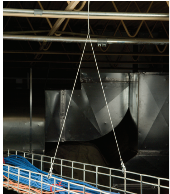
Figure 1: Speed Link SLK with Y-Hook holding wire basket tray
