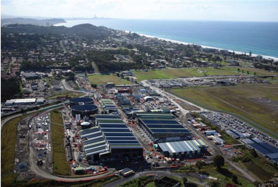
LENTON® FORM SAVER was used in the concrete construction of the Gold Coast Desalination Plant's pre-treatment building filter and flocculation tanks, residual treatment tanks and drum screen tanks.
