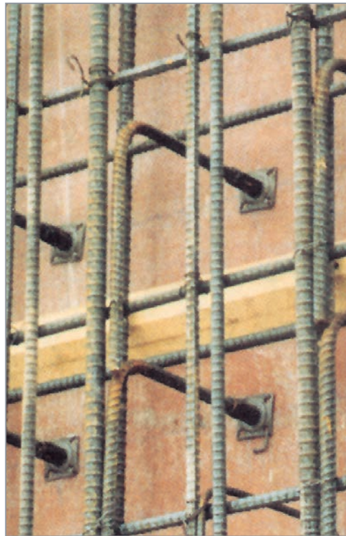
Instead of drilling, simply nail the Form Saver onto the form.
